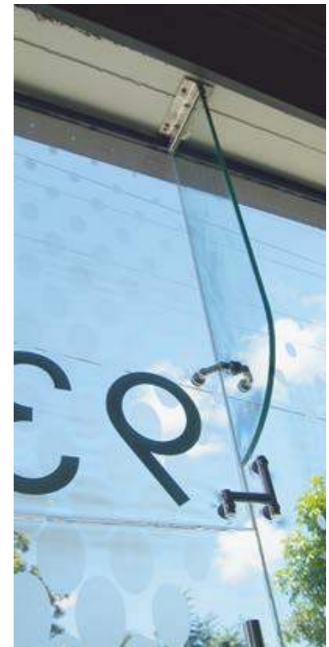
Typical cantilevered fin with bolt through back to back stainless steel head mounted fin bracket.
