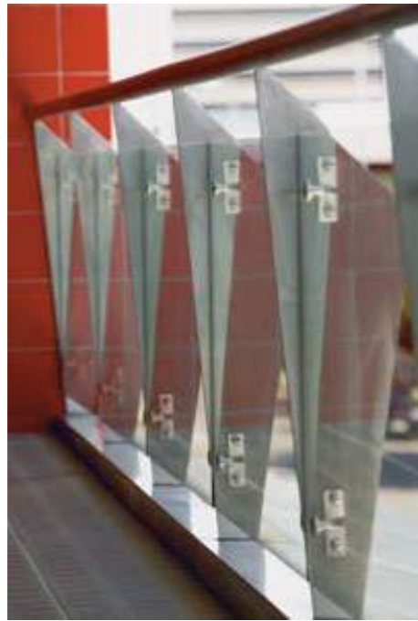
Spider fixing 2 edge supported.
