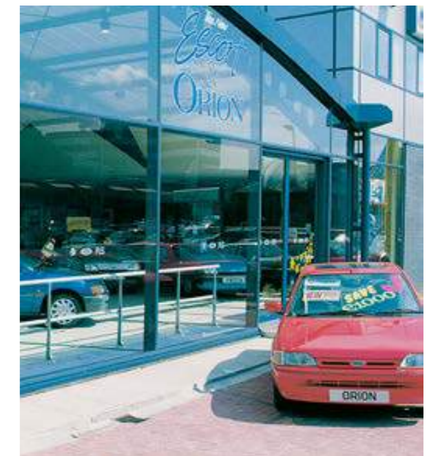
The top half of this shopfront is ordinary glass and anti-reflecting glass is glazed in the bottom half.
