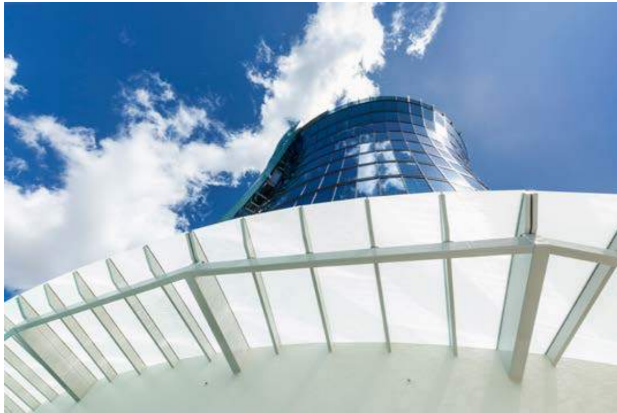
TW image printed with 17.52mm clear toughened SGP laminated - Riley Hotel Cairns
