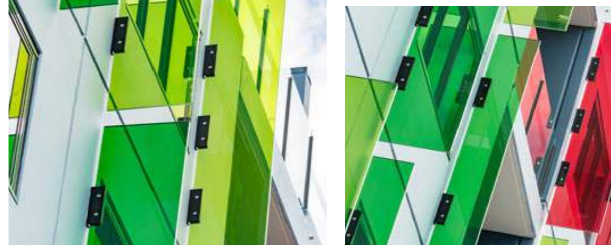
Custom laminated 17.52mm heat strengthened glass panels with Vanceva®coloured interlayers - Baxter St Apartments
