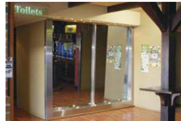
Laminated one way mirror – Subject side view from outside of men's restroom, lighting maximised to prevent see through.
