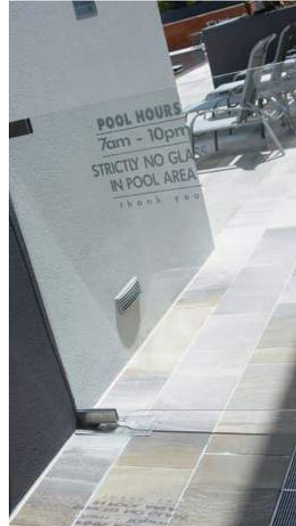
Frameless 12mm clear toughened pool gate with top/bottom corner patches and floor spring.
