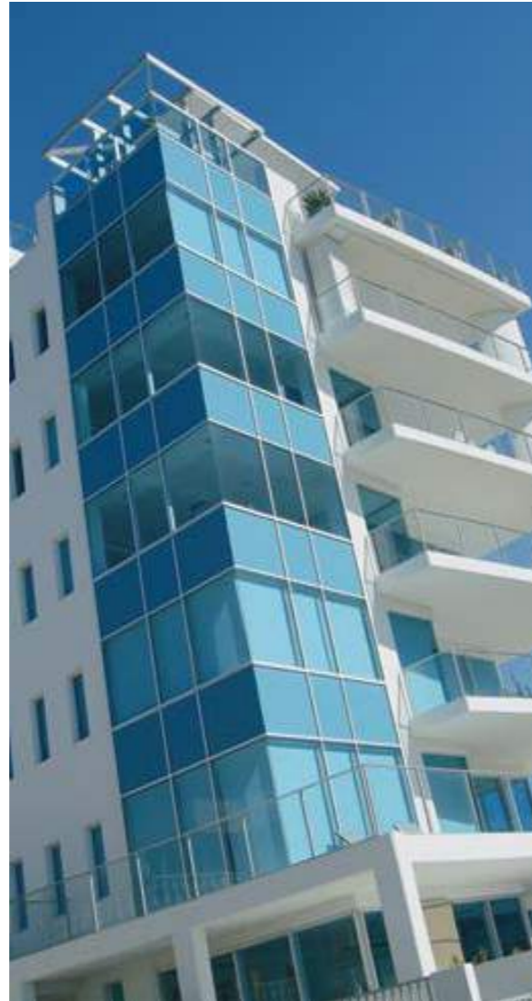
6mm Dark Blue vision glass with contrasting coloured spandrel glass
