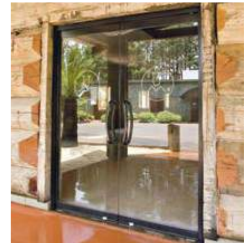
Type A top and bottom rail toughened entry doors.
