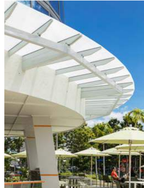
ImageTek™ Design custom image printed with 17.52mm clear toughened SGP laminated glass - Riley Hotel Cairns
