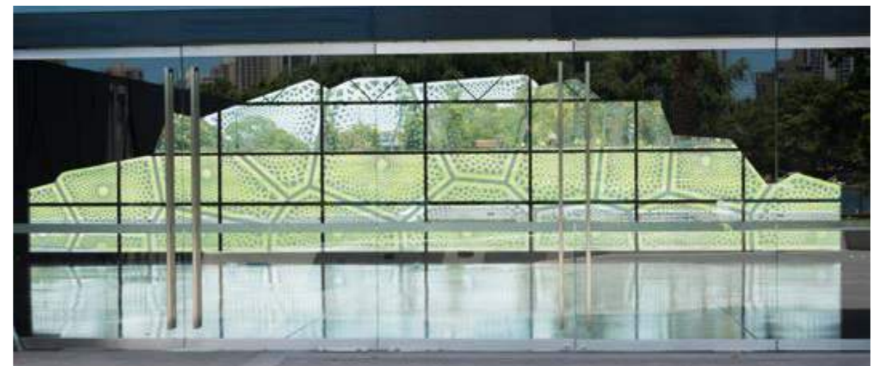
ImageTek™ Design custom printed image with 9.52mm SOL-XT Neutral 44 toughened laminated glass - Gold Coast Cultural Centre
