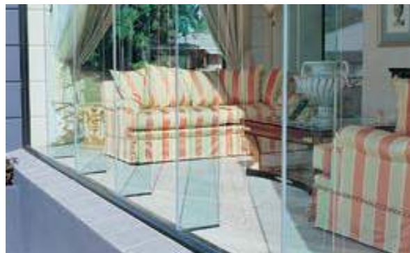
Single tier shopfront with full height supporting fin.
