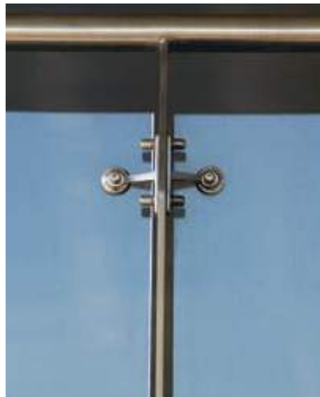
Close up detail of spider fixing.
