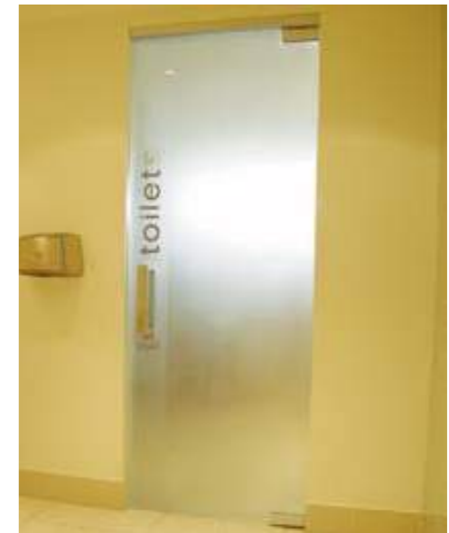
Type C top and bottom corner patch toughened entry door.
