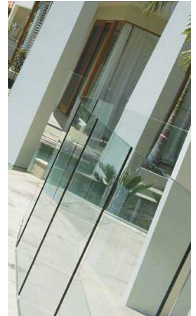
12mm clear toughened glass bottom grouted cantilevered.
